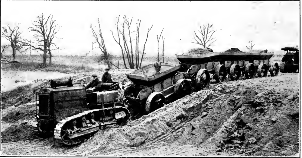
HOLT CATERPILLAR TRACTOR HAULING TROY TRAILERS IN THE CONSTRUCTION OF THE VICTORY MEMORIAL DRIVE BY THE BOARD OF PARK COMMISSIONERS OF MINNEAPOLIS, MINNESOTA
